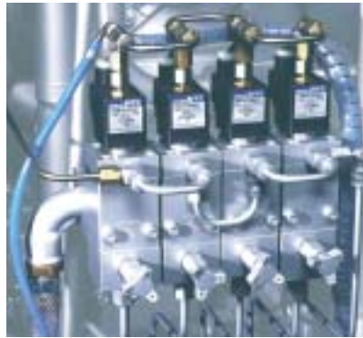
Automatic Condensate Drains
